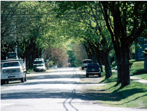
Figure X. The photo above shows a traditional street in Vancouver, BC where infiltration occurs in the crushed stone parking strips straddling either side of a 15' paved two way travel section.
