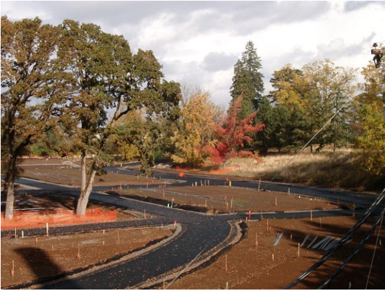
Figure X. The streets in the foreground are actually lanes paved with 13 ft (for fire access reasons) pervious pavement and crushed stone verges as described in the text.
