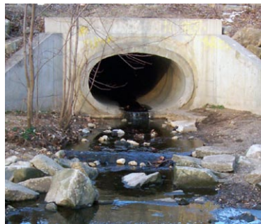
Figure X. A typical stormwater outfall seen here at a time of low flow. During high precipitation events the force of the water is enough to move boulders.
