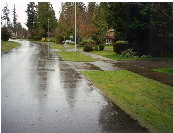
Figure X. This photo, taken in the Amble Greene Community of Surrey, BC, shows how in the absence of curbs rainwater can be directed to depressed boulevards where it is infiltrated into the soil.
