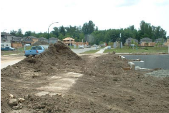
Figure X. Topsoil, preserved from the initial site grading, is returned to residential lots at the East Clayton development in Surrey, BC.
