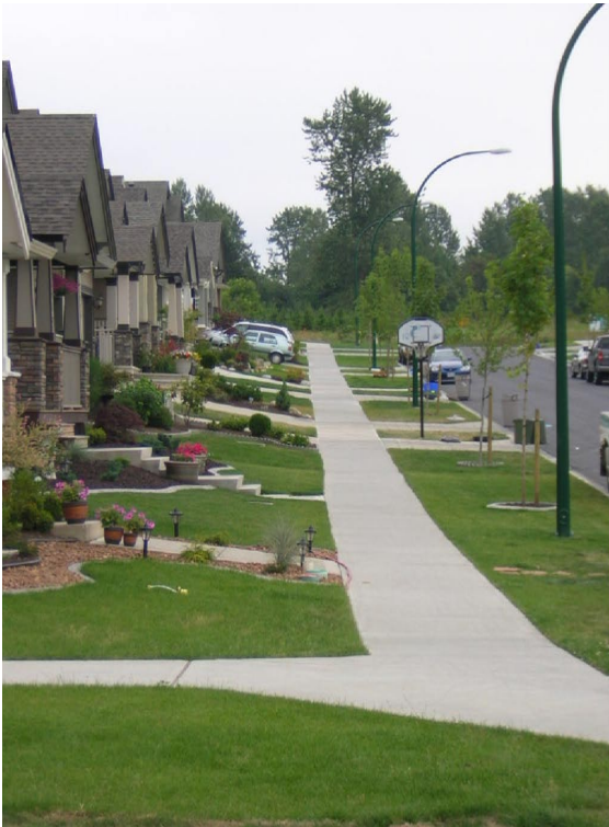
Figure X. The photo above, from East Clayton, Surrey, BC, shows slotted curbs that direct water into depressed boulevards
